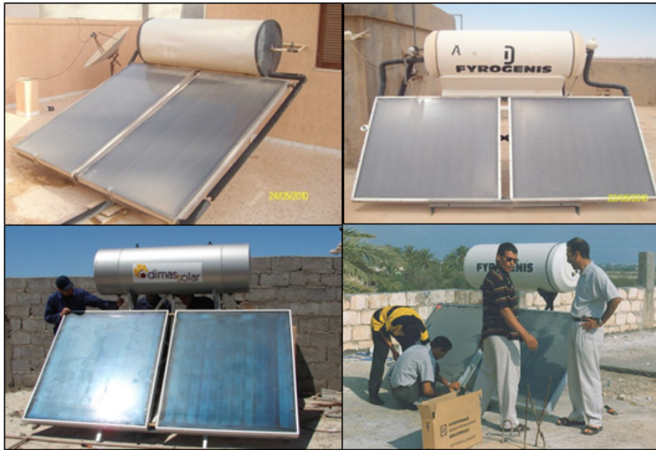
Figure (13). Solar water heaters installation by CSERS
